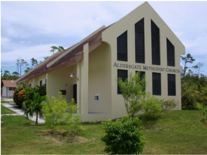
Hurricane-strengthened Aldersgate Methodist Church and School
