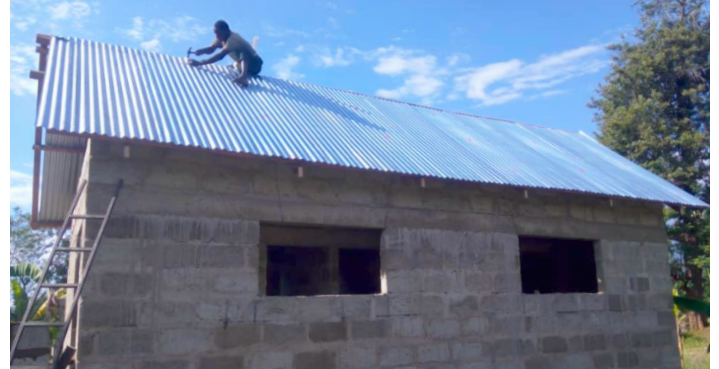
Roofing the Girls' Toilet Block of Lyasikika Secondary School
