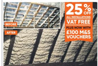
Typical example of a Roofsure Pitched roof Installation, Insulation is applied between the structural timbers to a breathable membrane.
